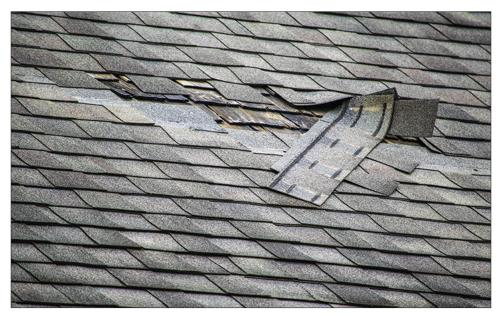
find dark streaks or moisture in the attic may discover that water is penetrating the roof underlay. Water often comes in around chimney flashing. Other water signs are blistering and bubbling in walls.
